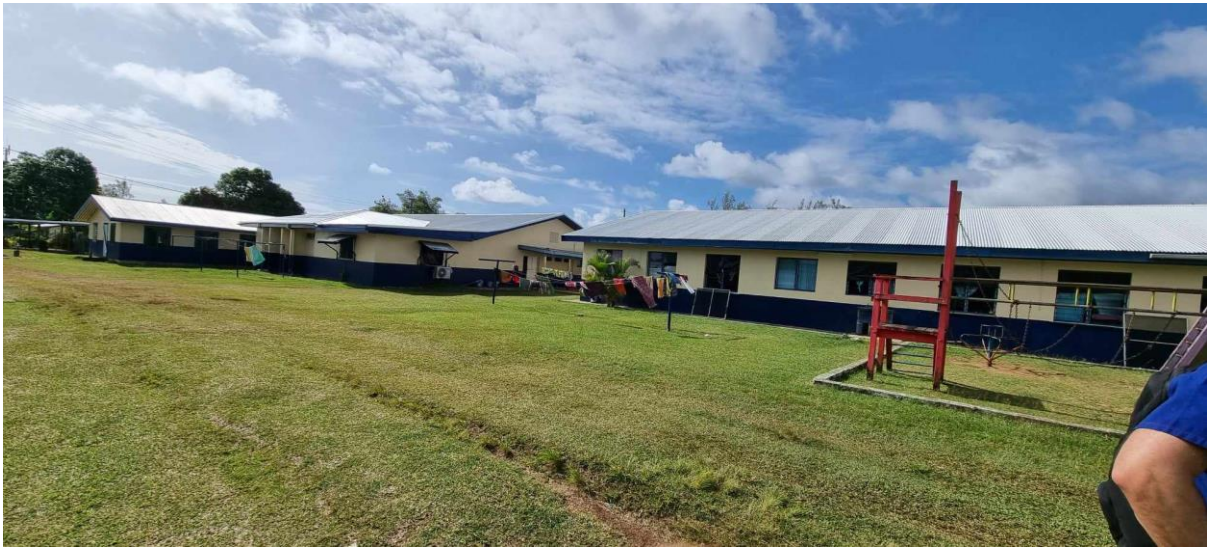
The rear of Northern Provincial; paediatrics ward to the right and obstetrics ward to the left
